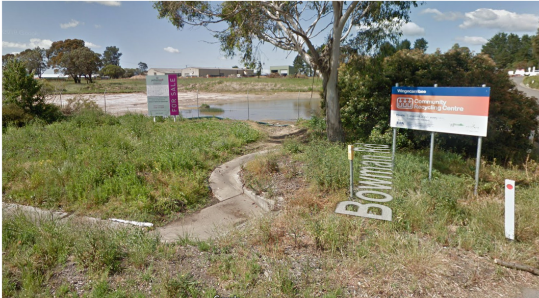
Figure 3.5: View of headwall inlet at Berrima Road and Bowman Road, including wet infiltration system at 1 Bowman Road (Google Maps)
